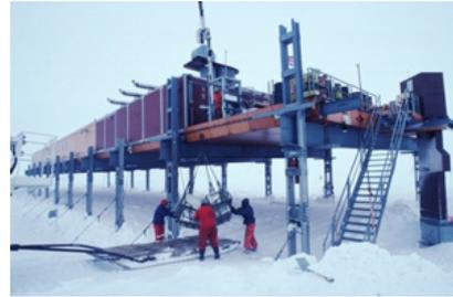
keep the structure square and true, each of the legs is braced outward with a stainless steel wire. It is vitally important that the wire tension limits are not exceeded as the temperature falls.
